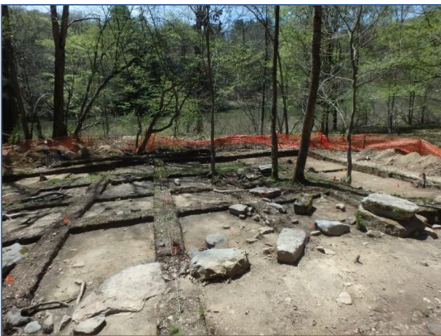
Excavation of former house site (Feature 1) in progress with support stones visible.
