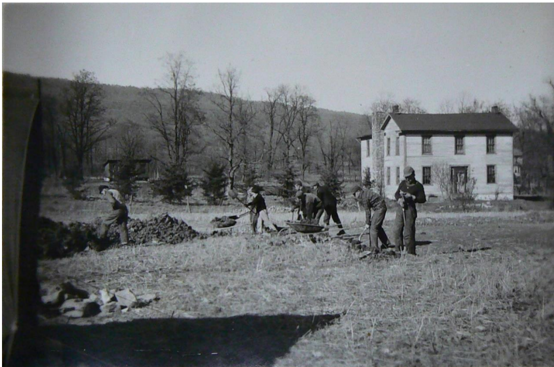
1939 excavation photo. (Image courtesy of Janet Johnson, PHMC)
