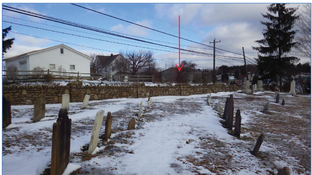
Gilmore to Welsh Hill Road project. A view of old Friedens Cemetery looking toward the area across Route 281 where a retaining wall (at arrow) was removed.
