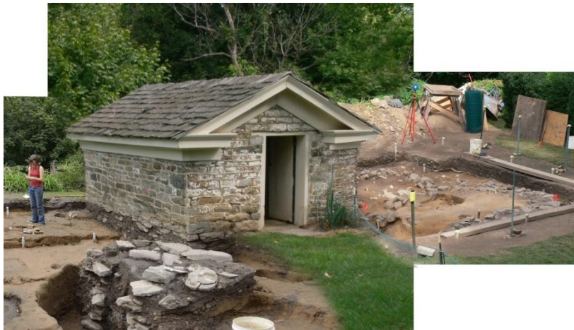
Figure 3 Well, milk house and smoke house foundation image.
