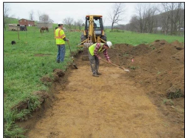
Figure 2. Monitoring machine-assisted removal of plowzone and shovel-shaving top of subsoil.
